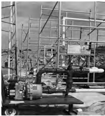
Centrifugal pumps with pressure release valve
