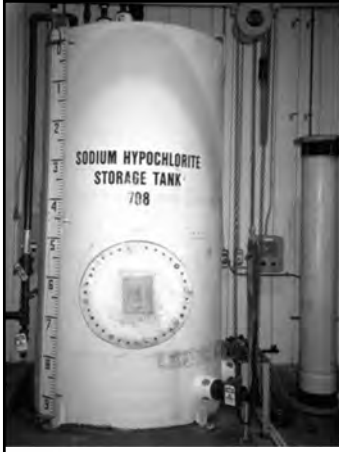
Sodium Hypochlorite Storage Tank
