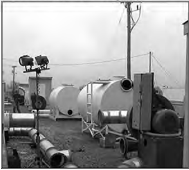
Activated Carbon Units to Remove Contaminant in the Vapor
