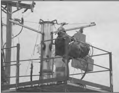
Stack emission test
