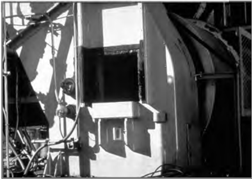
Incinerator Primary Chamber
