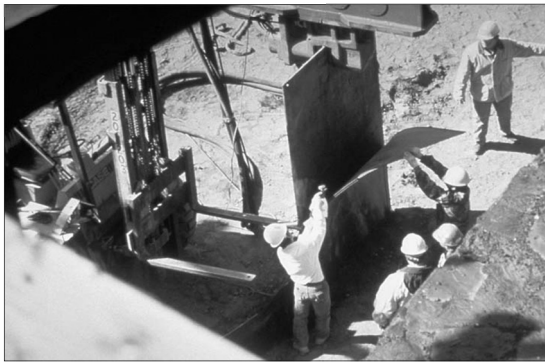
HDPE Sheet Piling
