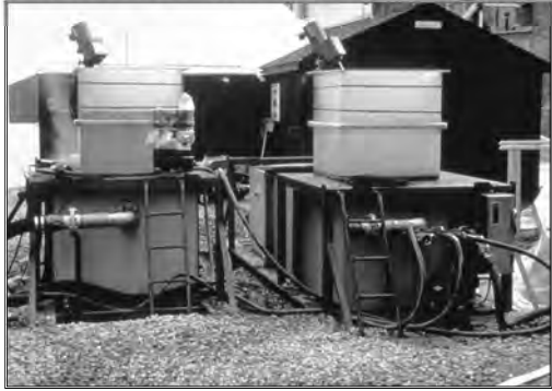
Incinerator Scrubber with Mixing Tanks
